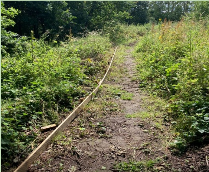
PFP 9 Penyffordd Surfacing work with stone to improve access.
