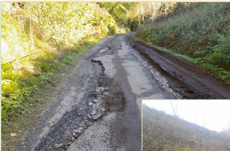
Footpath 21 Holywell Pilgrim's Way repair to eroded surface using tarmac.
