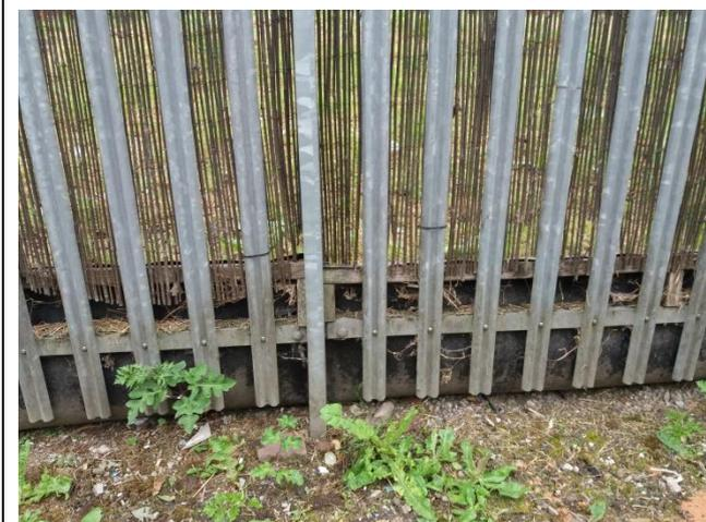
**Photograph 6:** Existing amphibian exclusion fence in place at base of perimeter fence of Site
